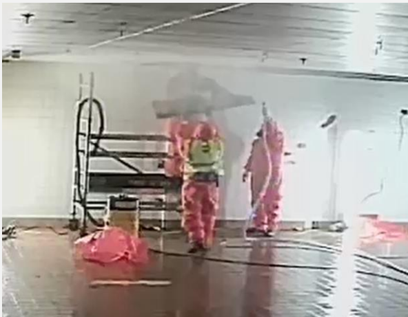
07/08/23 08:15 Removal of initial tiles
